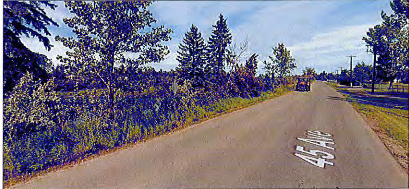
Figure 7: 45 Ave between the river and subject property. Note narrow width of riparian strip, lack of shoulders, lighting, and curbs. (Google Maps accessed 2022 22)
